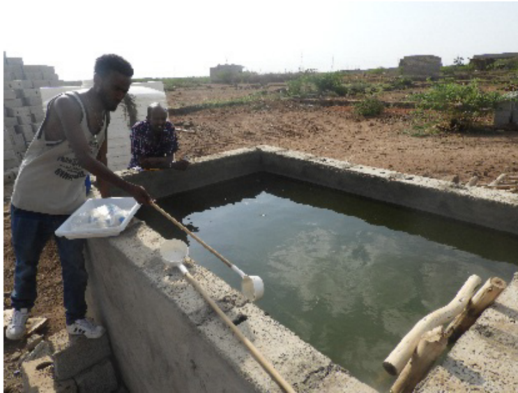
Figure 2b. Concrete cistern in Ethiopia
